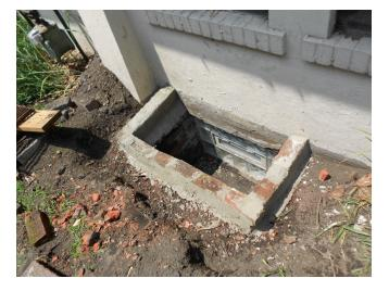
There was an exterior basement window that had just been back filled with dirt, the window was broken and the frame crumbling from rust. In order to reduce the moisture getting into the basement we had the window replaced with glass block.
