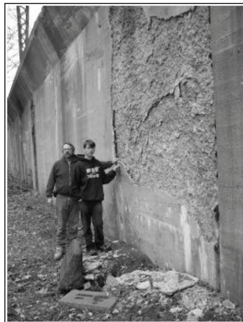
After two years, a railroad claimed this wall. Wyane and son Jeffrey Rhine, of the East Cleveland Township Cemetery Foundation, with crumbling railroad embankment wall near gravestones.
